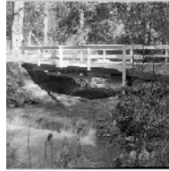
Stream (ی) and Bridge
